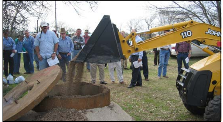
Well Plugging Demonstration- January 26, 2005
